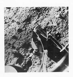
Cover Photo: Surveyor VII photo showing the surface sampler transporting the alphascattering sensor head to the second lunar sample to be analyzed, the round rock indicated by the arrow.
