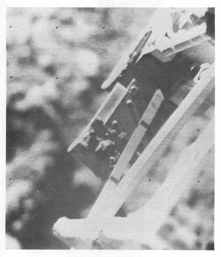
Figure 5-22. — Fragment adhering to surface-sampler magnets after contacting lunar surface (day 020, 14:57:46~GMT).
