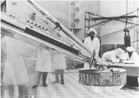
Fig. VII-13. Magnet assembly before flight. The magnetic bar is on the left; the nonmagnetic control bar is on the right. Magnetic flux along the pole edges is about 600 gauss. The control bar has flux readings of less than 0.1 gauss over the surface of the bar. Dark "S" on magnet side indicates the south pole. (a) Footpad 2 assembly. (b) Footpad 3 assembly.
