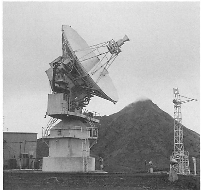
Fig. V-10. DSS 72 30-ft antenna system at Ascension
