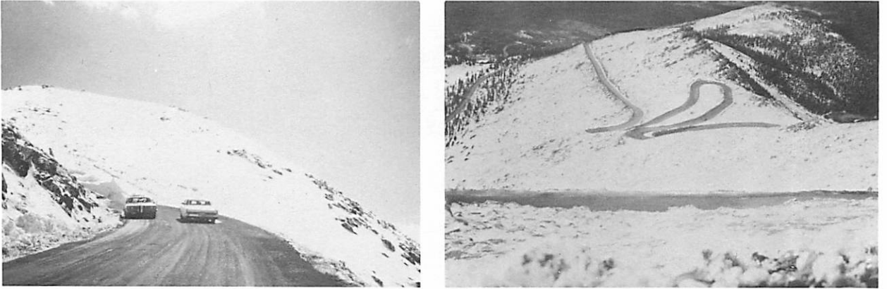
Fig. 26 Views of road near 13,000 ft level, not safe except in summer.
