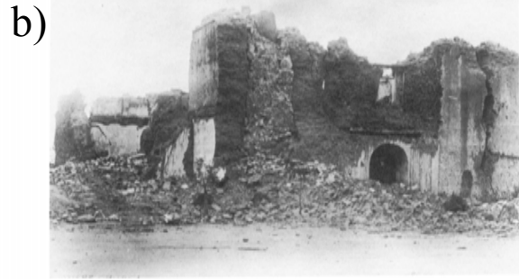
(top) Church in Bavispe, Sonora, after 1887 earthquake. (bottom) Earthquake destruction in Bavispe. —Arizona Historical Society, Tucson.
