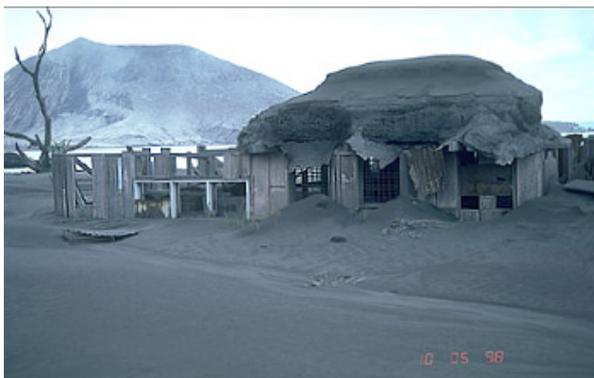
Figure 2: This house was damaged by a heavy load of ash that accumulated on the roof during the eruption of Rabaul Caldera in 1994
