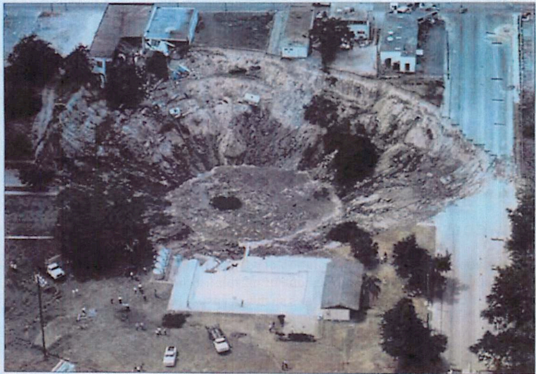
Figure 62. Spectacular, sudden collapse of the land surface commonly accompanies the formation of a sinkhole, such as this one that formed at Winter Park, just north of Orlando, Fla., in 1981.
