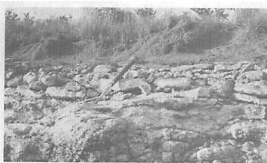
Figure 3-12. Caliche plates formed on West Texas caliche.
