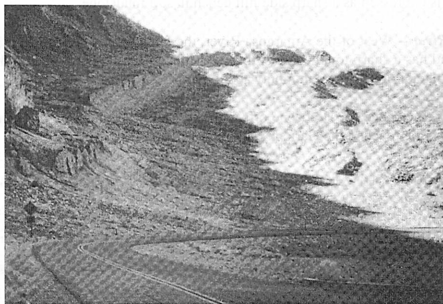
Fig. 7 – View to the southwest from Badwater showing fault scarps on the Badwater alluvial fan. Scarps that are erosionally enhanced identify the approximate location of the fault that has offset fan surface. Two fault scarps join to form a single scarp on the horizon. (From Wills 1989)
