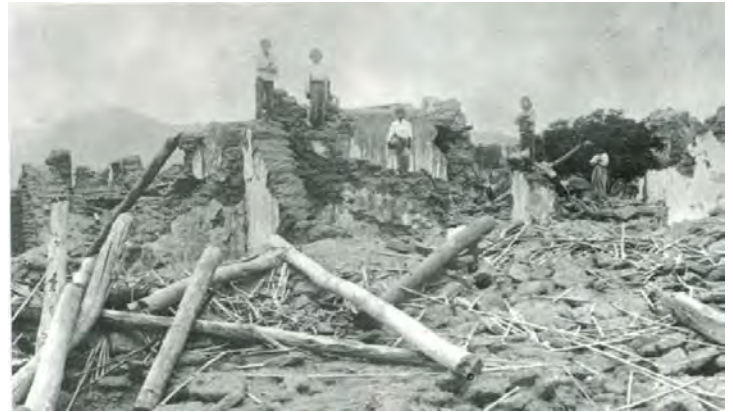
Figure 5. Damaged buildings in Bavispe, Mexico which lies close to the Otates fault [9].
