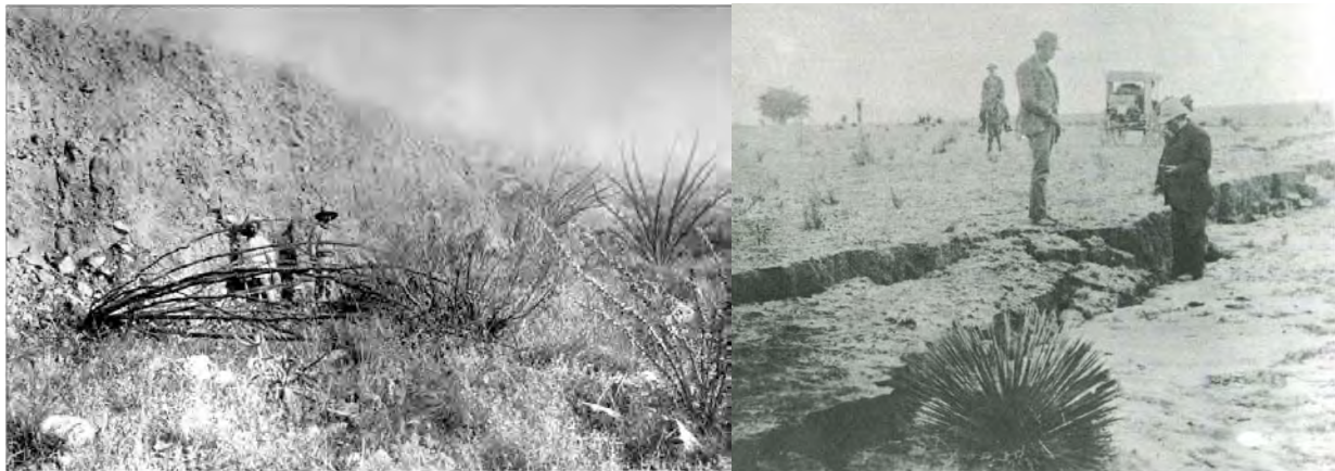
Figure 6. Historic 1887 photographs of fissures formed by the earthquake [9].
