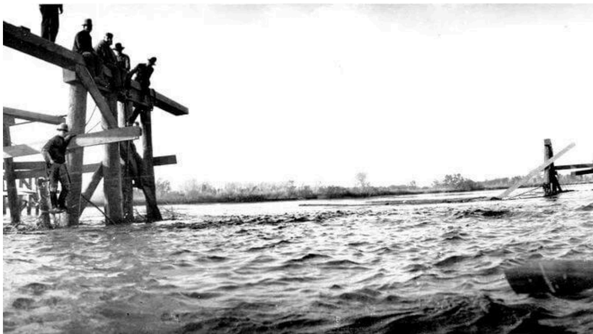
Figure 2. They took the Chevy to the Levee but the Levee was NOT dry. Attempts to stem the floodwaters sometime between 1905 and 1907. (Photo courtesy of the Salton Sea History Museum via The Imperial Valley Press.)
