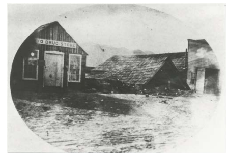
Figure 3: A collapsed adobe structure between two undamaged wood-frame structures.
