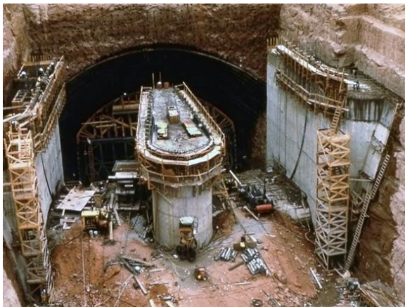
Glen Canyon Dam Spillway Construction - 1963
